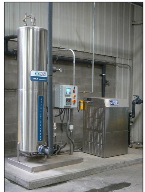
Figure 1: The Pacific Ozone Horizon Series integrated ozone system is the heart of the plant-wide ozone loop.
